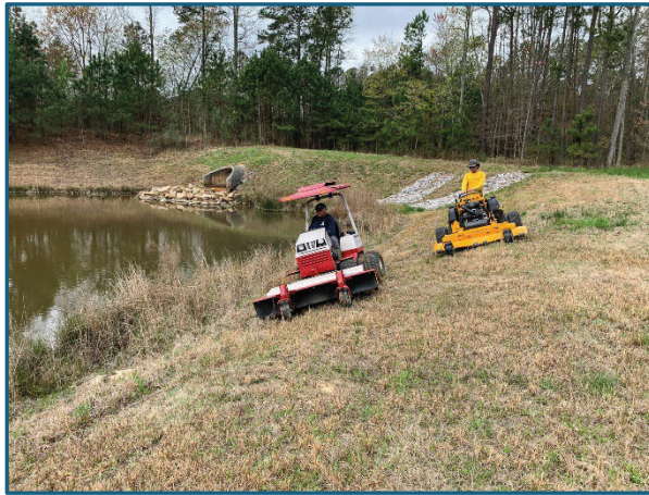
Figure V.2: Example Stormwater maintenance
